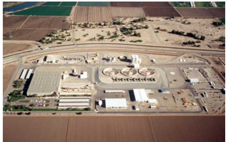
Figure 2: Yuma Desalination Plant, photo c/o www.usbr.gov.lr
