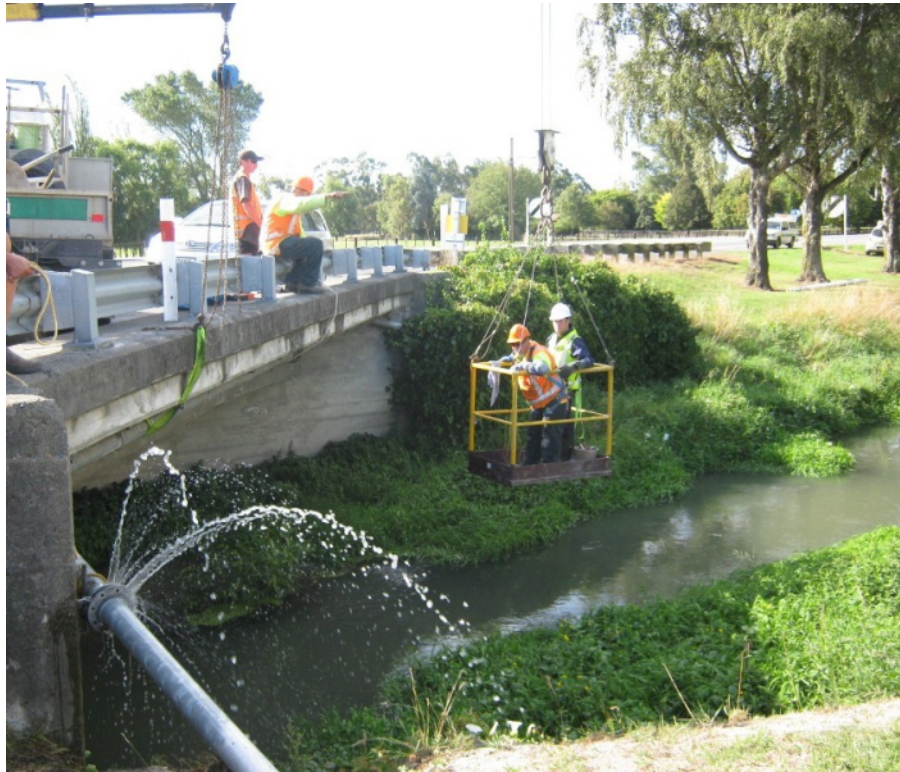
Photograph 3: Breaking Pipe at Tai Tapu
