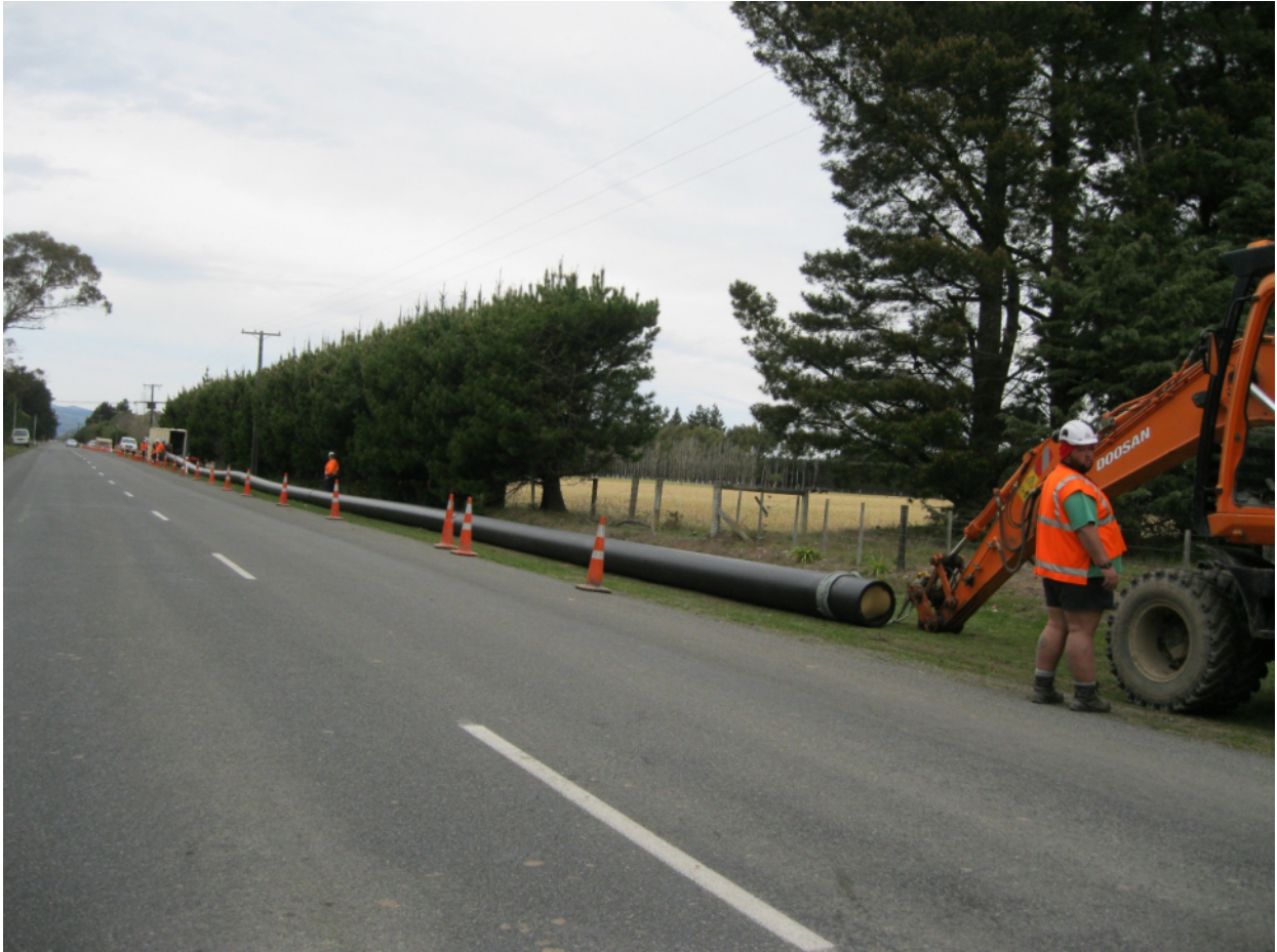
Photograph 4: Pipe installation as part of ESSS
