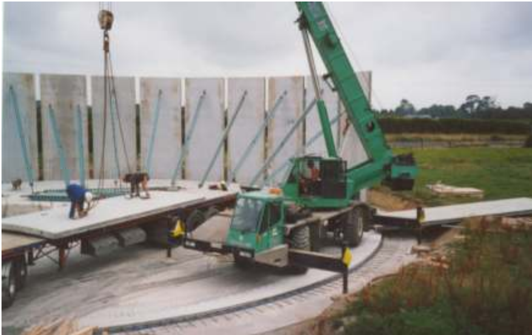
Figure2: Barrett Road reservoir under construction
