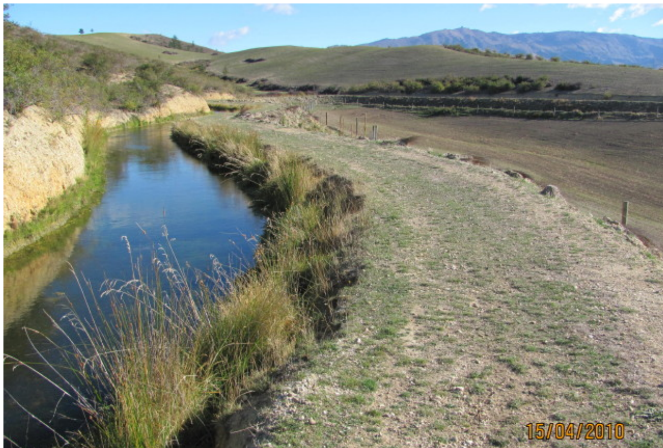
Photograph 1: Main race of Manuherikia Irrigation Scheme
