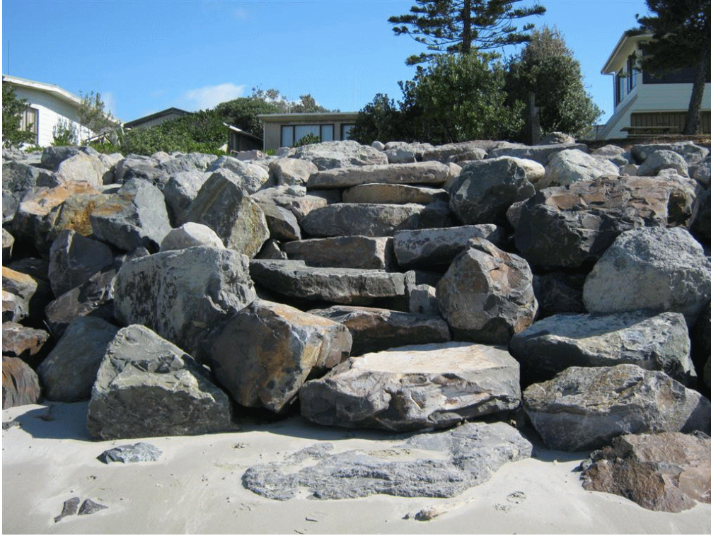
Photograph 10: Emergency Exit / Informal Beach Access 85 / 87 Shaw Road
