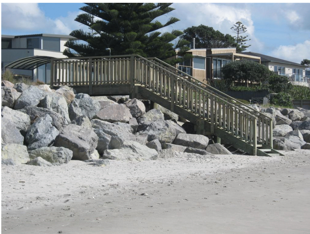
Photograph 9: Public Beach Access 21a
