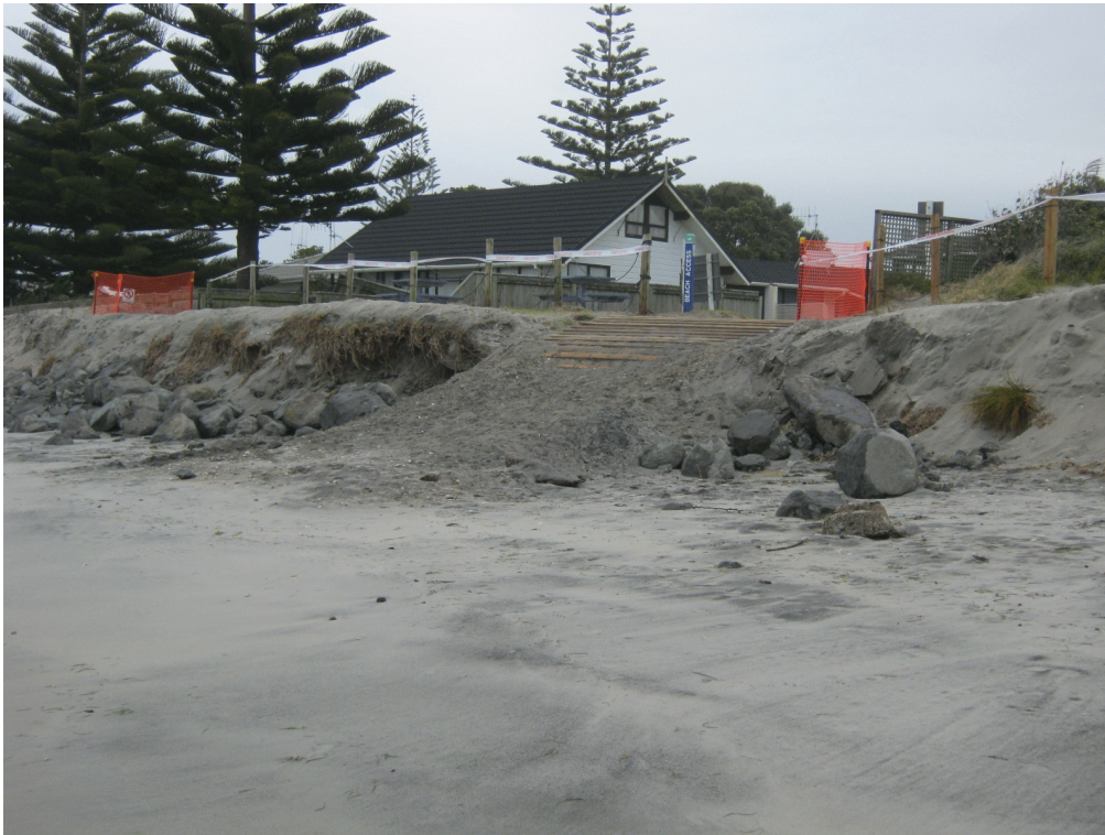
Photograph 8: Dune erosion at Beach Access 14 (inside work area)
