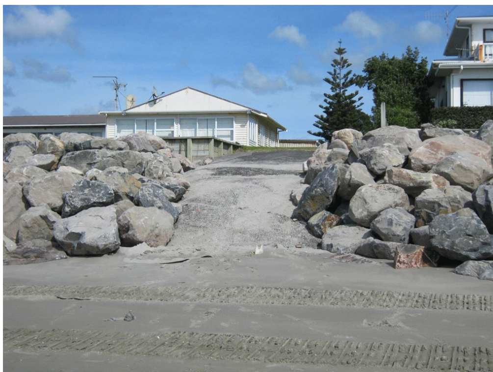
Photograph 11: Boat Ramp and finished revetment at 81 Shaw Road
