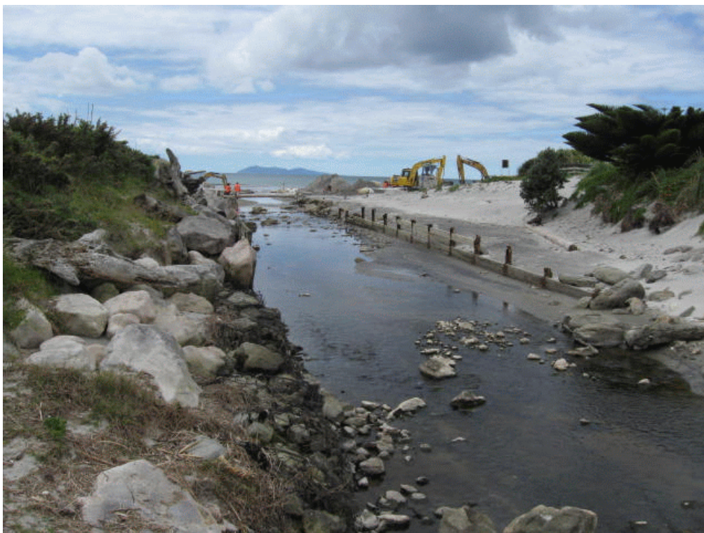
Photograph 1: Three Mile Creek during construction
