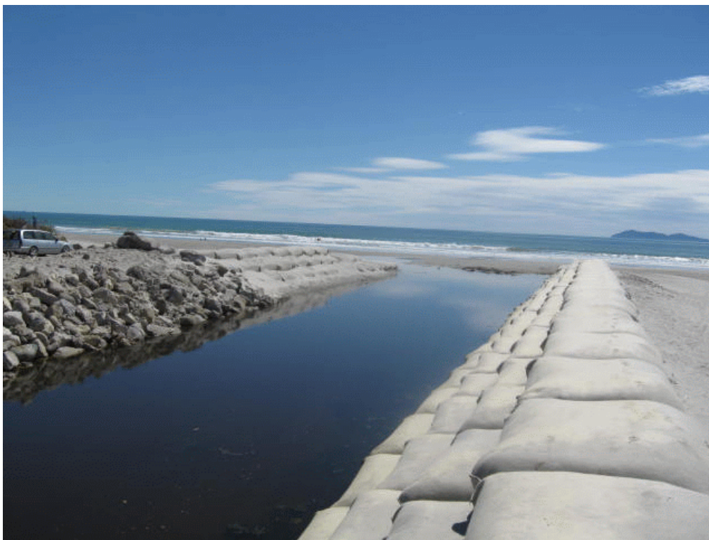
Photograph 2: Three Mile Creek after construction
