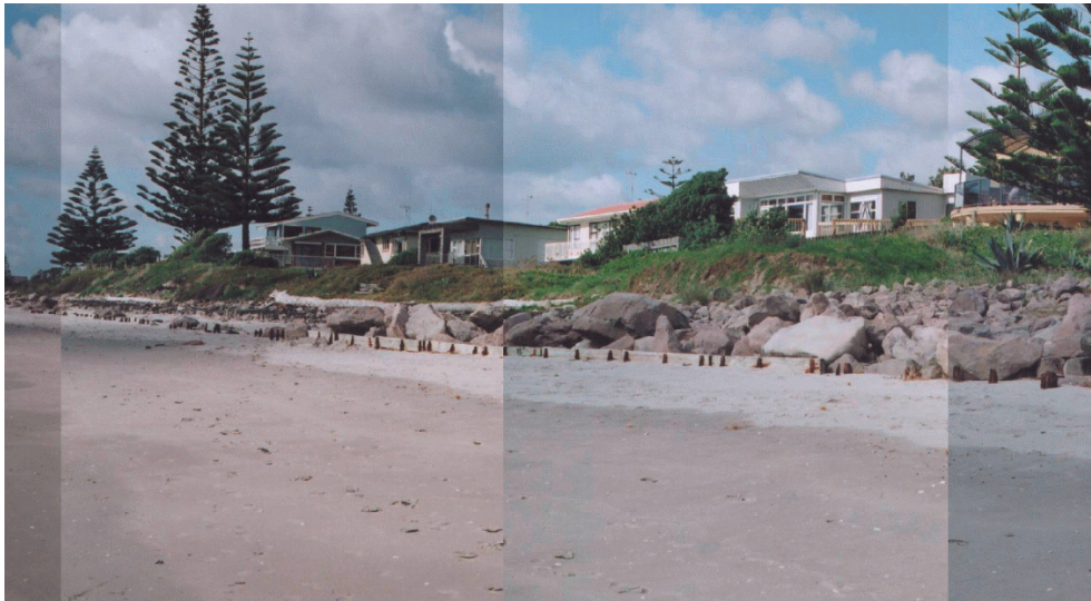
Photograph 4: The Loop before construction
