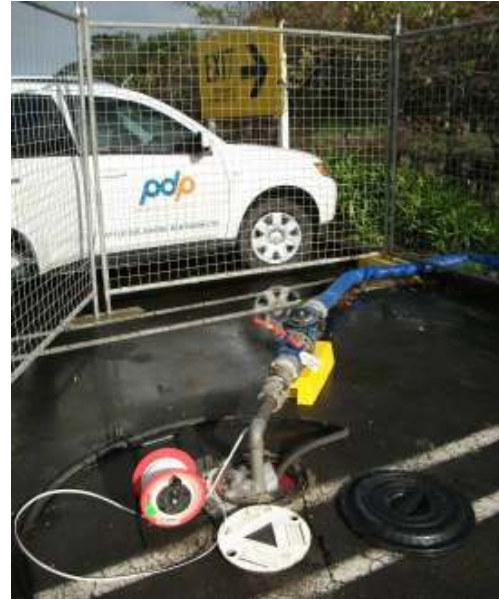
Photograph 2: Pak 'n Save pumping test: pumped bore DH950
