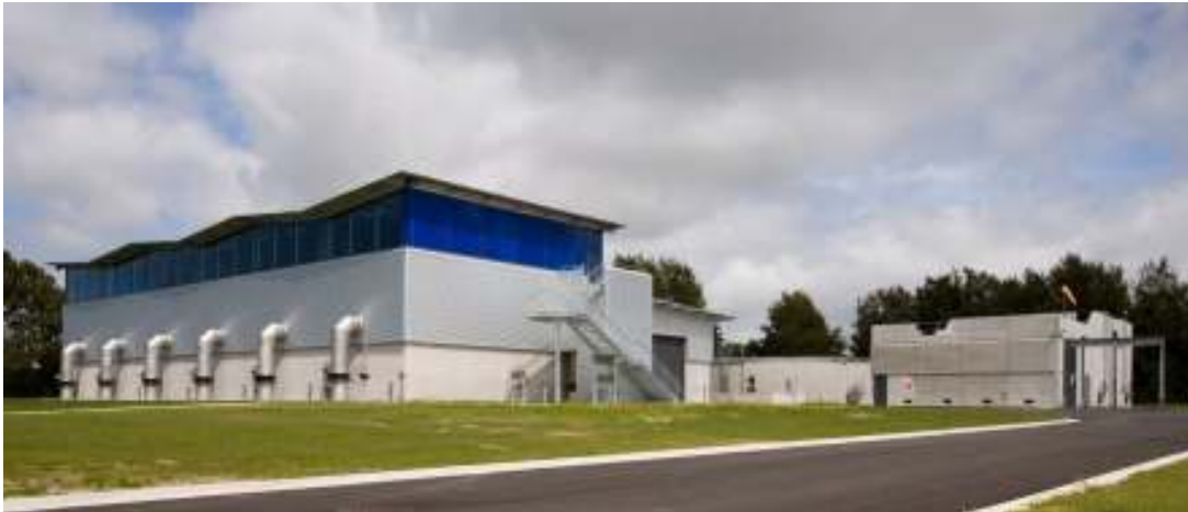
Photograph 1: Overall Upgraded Facilities
