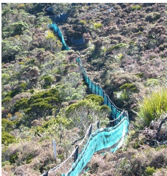
Figure 14. Silt fence installed prior to mining.
