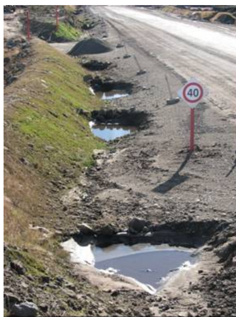
Figure 15. Roadside check dams at Stockton Mine.
