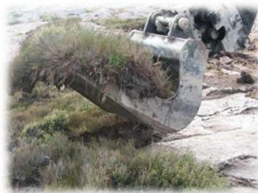
Figure 12: VDT bucket salvaging thin sods from pavement. The bucket has a cutting front edge and flat base
