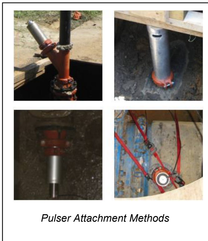
Figure 10. The various methods for attaching Acoustic Pulsers to Pipelines
