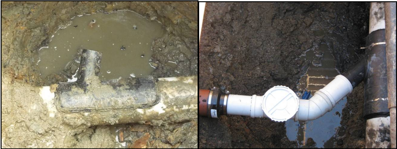
Photograph 1 and 2 – The lateral junction repair on the Progressive Plastics lateral
