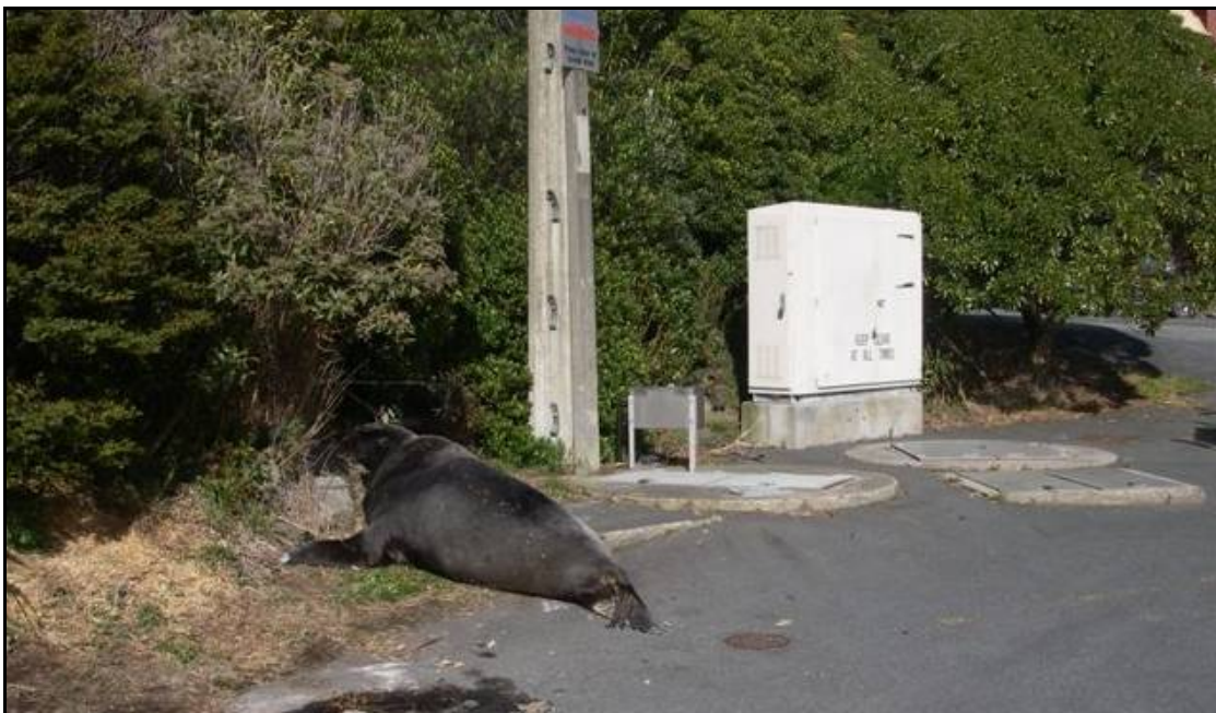
Photograph 13 – A large sea lion obstructing access to a pump station
