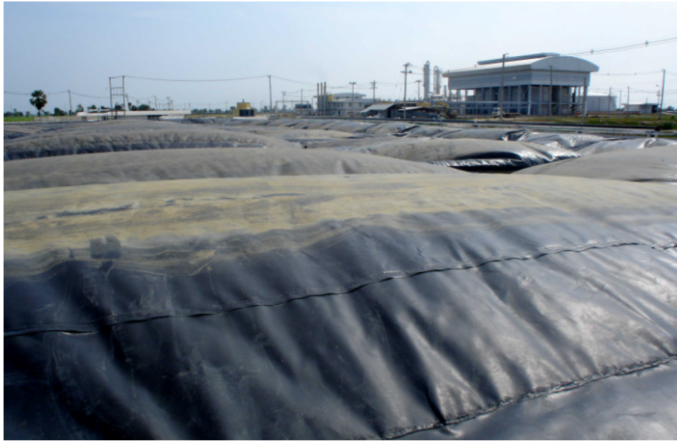
Figure 3: Overview of the mesophilic CIGAR™ digester system at Thai Agro Ethanol in Thailand (2005). This system treats 700 m 3 /day molasses distillery waste with a COD content of up to 200,000 mg COD/L.
