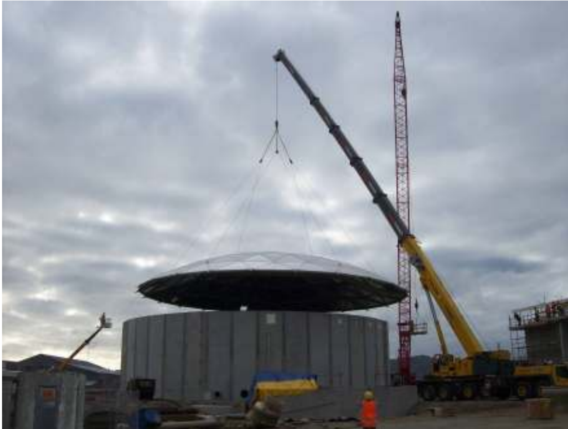
Photograph 3: Crane lifting BTF cover in place
