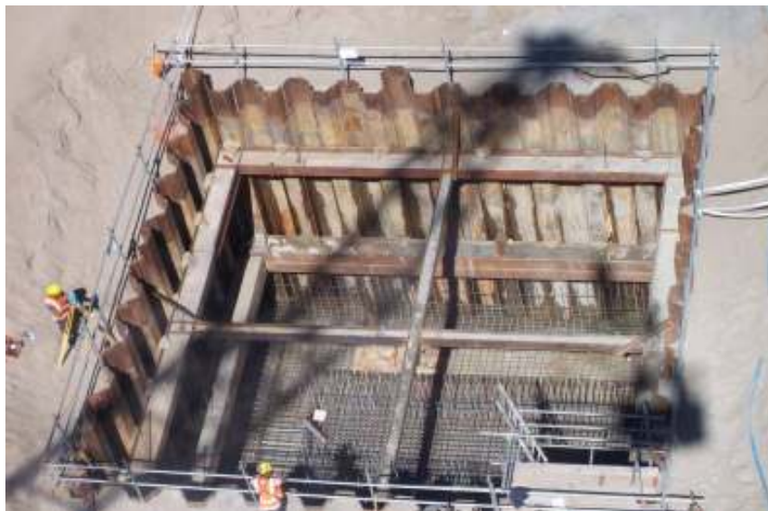
Photograph 1: Sheetpiling to Outfall Pump Station
