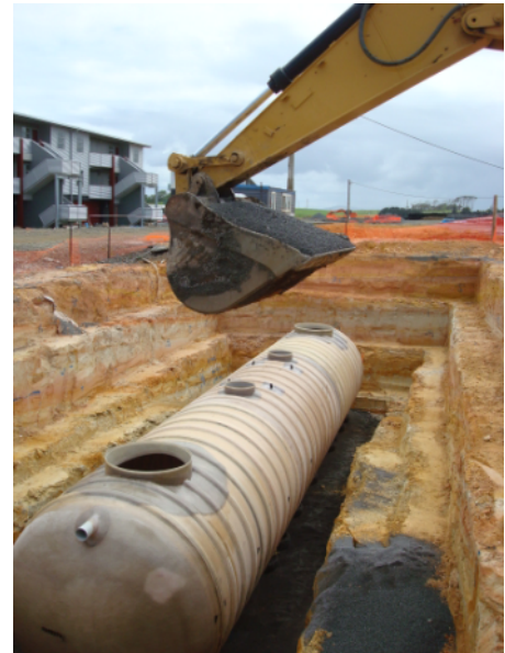
STEP tank installation
