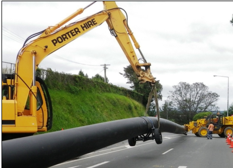
Photograph 3: PKS Polyethylene manhole being installed on pipeline SP202
