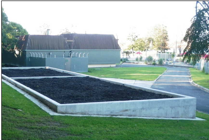
Photograph 7: Memorial Park biofilter with fan compound and existing pump station in the background
