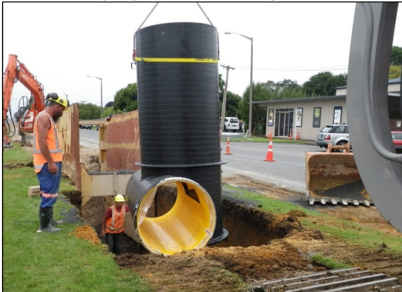
Photograph 3: PKS Polyethylene manhole being installed on pipeline SP202
