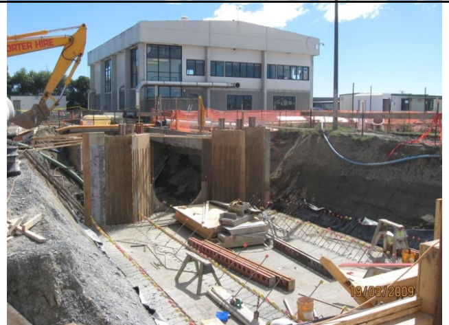
Construction of the Papatuanuku channel, March 2009
