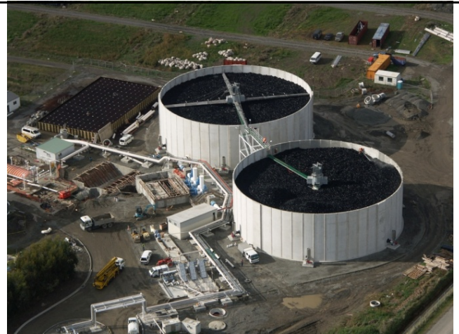
Plant under construction, May 2009
