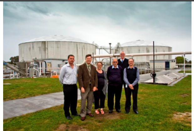
The HDC/MWH project team in front of the completed plant. Left to right: Matt Kneebone, MWH's Engineers Representative; David Fraser, HDC's Group Manager Asset Management; Rachel Landon, HDC's Wastewater Treatment Programme Manager; Bob McWilliams, HDC's Wastewater Treatment Plant Manager; Des Parkinson, MWH's Project Manager; Brett Chapman, HDC's Water Services Manager, October 2011
