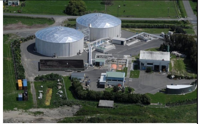
Completed domestic treatment plant with the milliscreen plant and outfall pump station, October 2011
