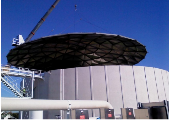
Installation of the geodesic dome covers, June 2011
