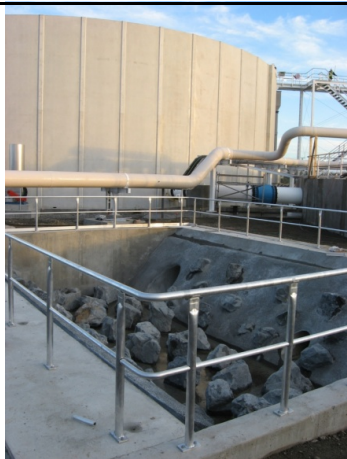
Completed Papatuanuku channel, June 2009
