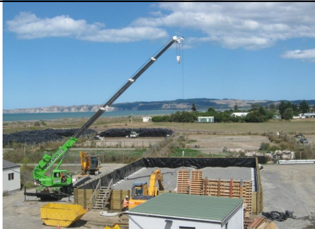
Bark Biofilter construction, February 2009
