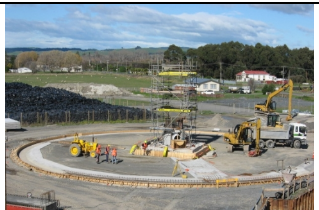
Construction of the BTF tanks commences, August
