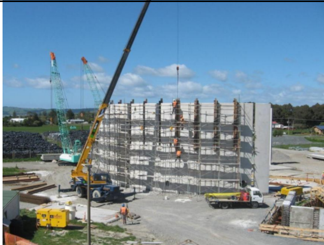
BTF tank panel construction, October 2008
