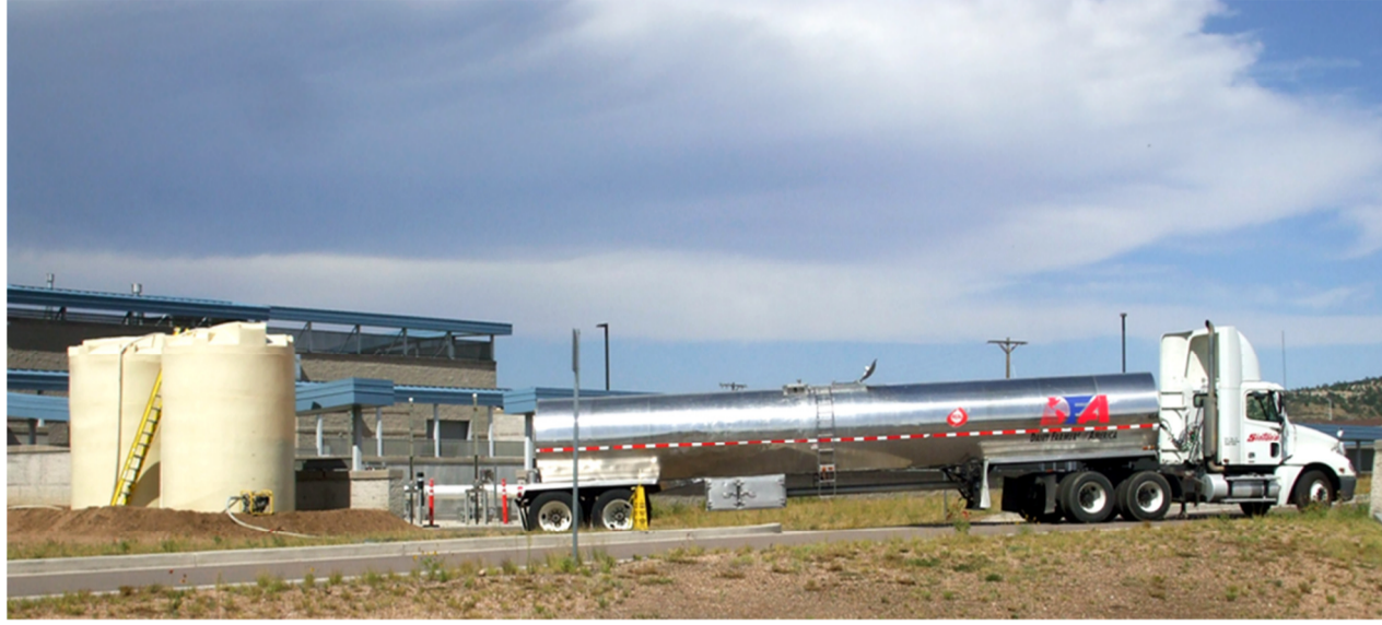
Figure 2. Acid Whey Delivery to Temporary Storage Tanks
