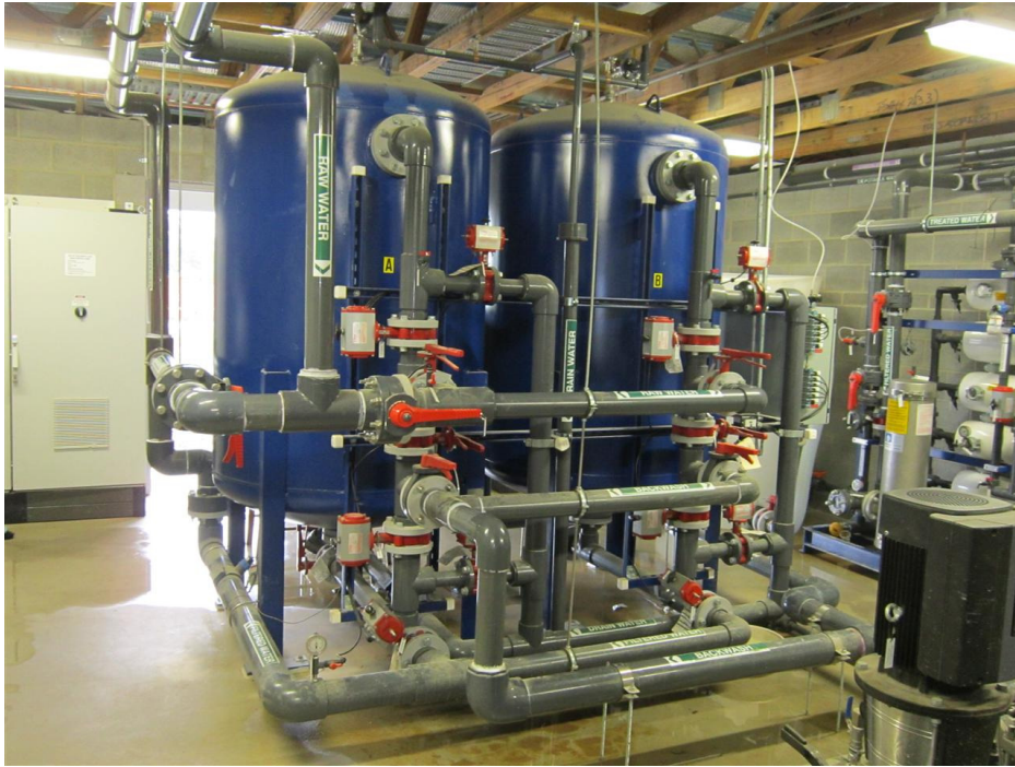
Photograph 3: Skid Mounted RO Plant
