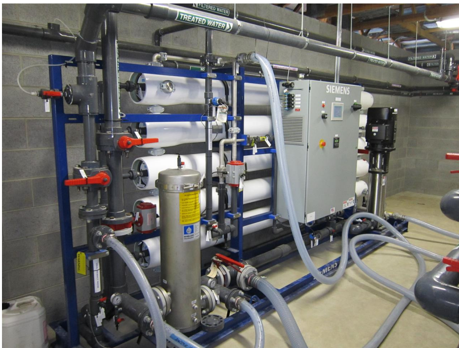
Photograph 3: Skid Mounted RO Plant
