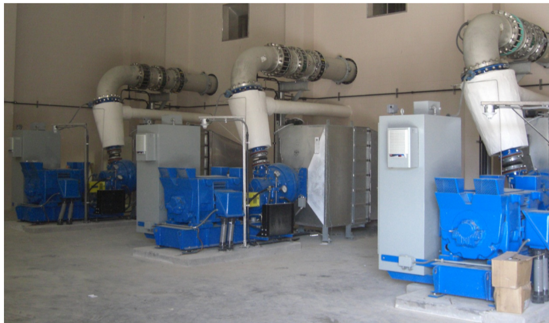
Figure 10. Case Study Blowers at 90 Percent Complete Installation
