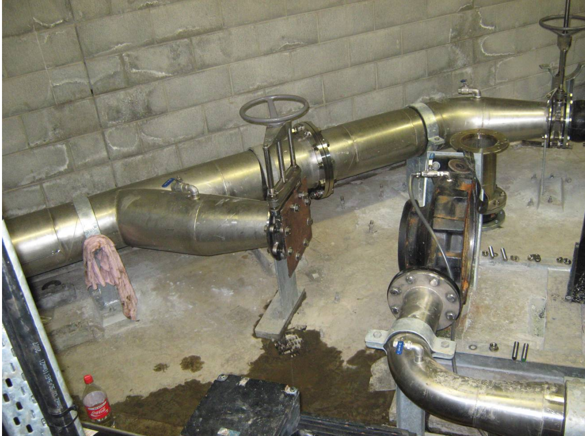
Photograph 19: Work on pump 2 showing pump & pipework removed
