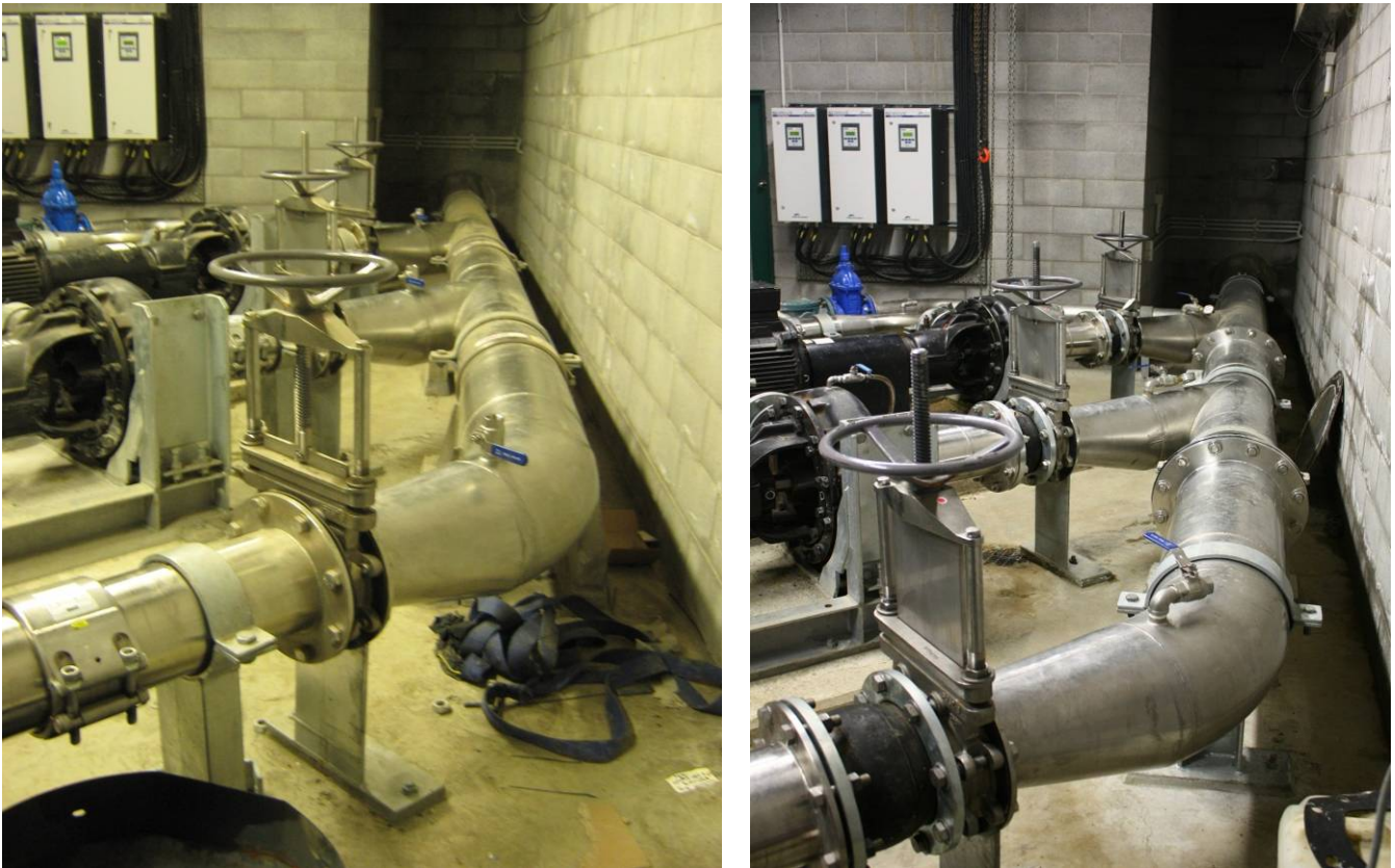
Photograph 4: Before and after header pipework configuration
