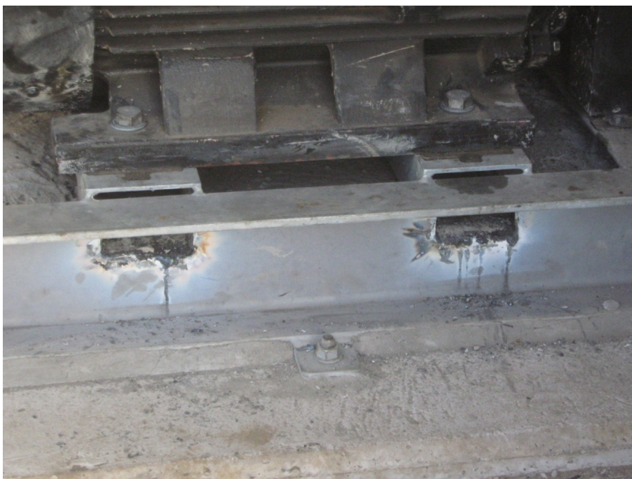
Photograph 11: Pump 3 chassis showing access slots cut to enable motor adjustment.
