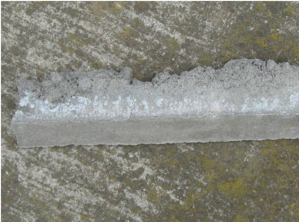
Photograph 16: Sample of original dry pack from under pump 3
