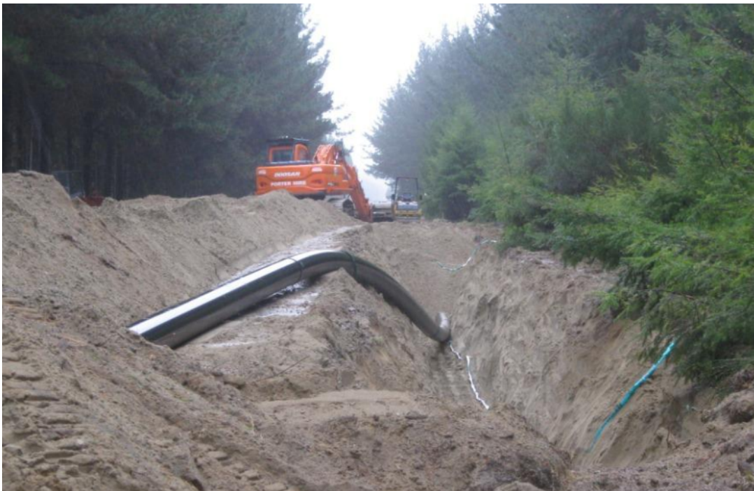
Photograph 5: Pipeline installation on Rabbit Island
