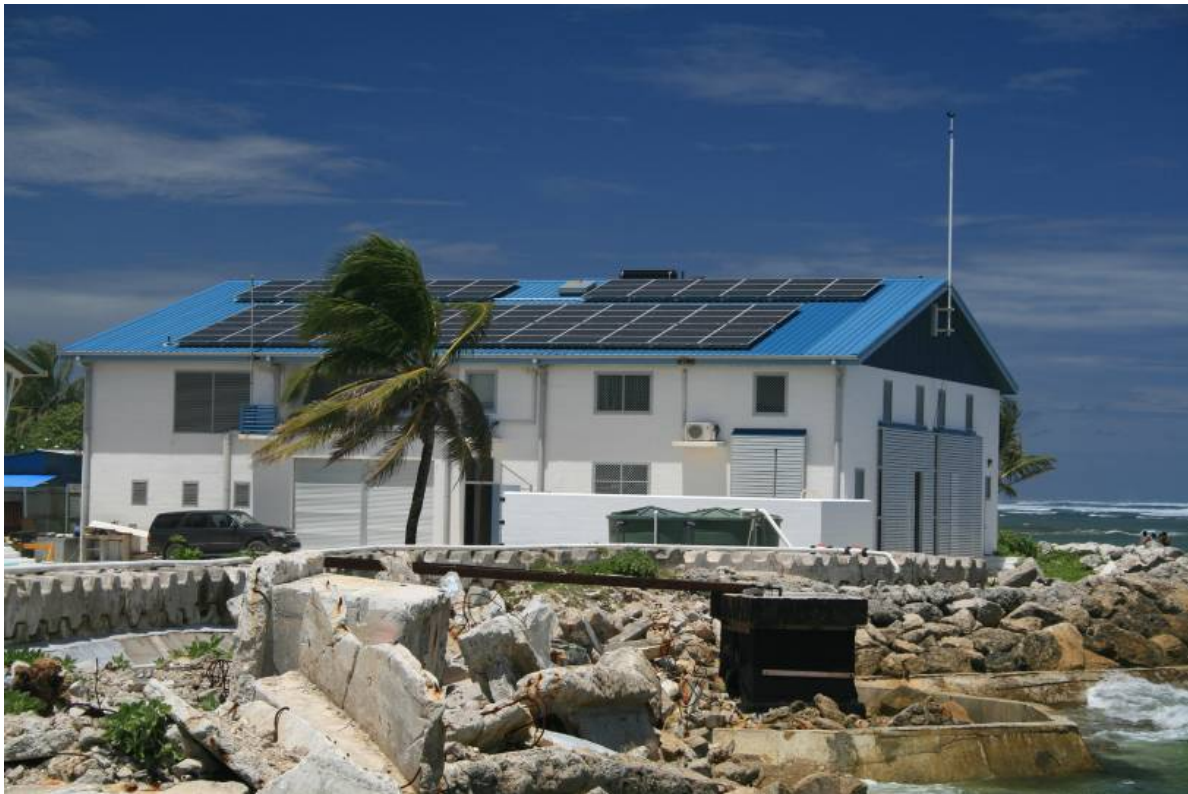
Figure 7: Utilities building showing PV panel installation.
