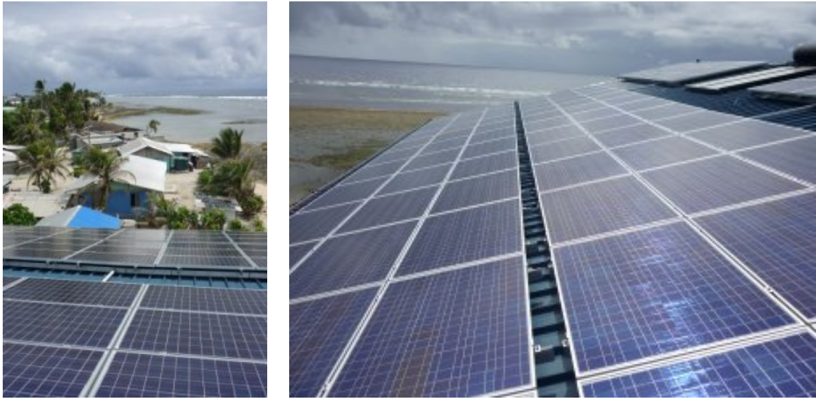
Figure 6: PV panels installation
