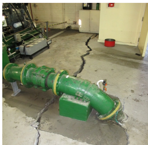
Photograph 1: Huntsbury 1 Floor Slab and Typical Pump Station Floor Slab Damage
