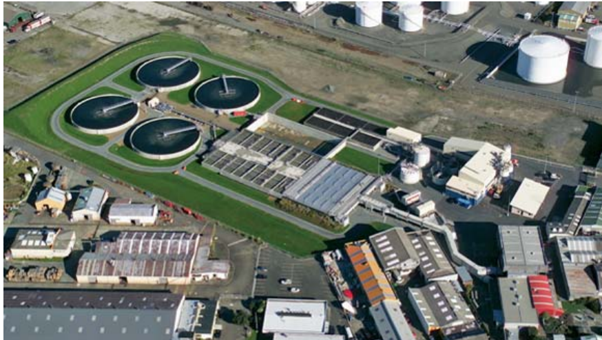
Figure 14 Overhead Photo of Seaview WWTP, Lower Hutt, Wellington, New Zealand. The Biological Process with the four (4) Secondary Clarifiers, are clearly identifiable on the left of the photo.
