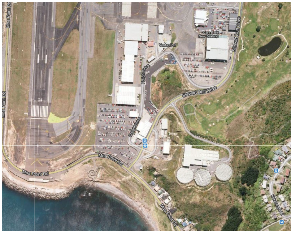
Figure 16 Overhead Shot of Moa Point WWTP, Wellington, clearly showing the close proximity of the airport (runway) and houses.
