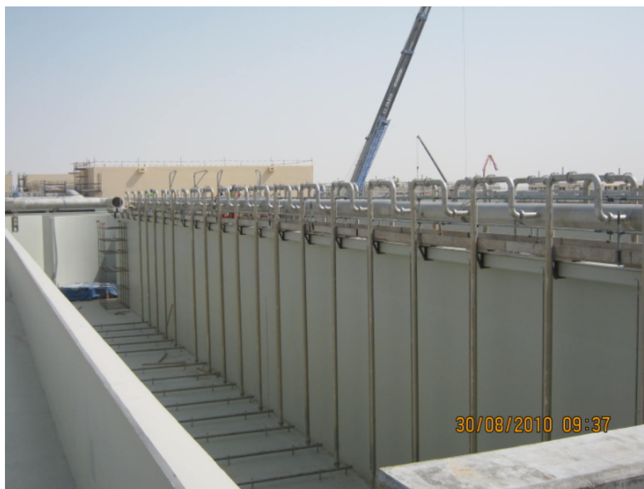
Figure 11 Wathba 2 WWTP Construction
