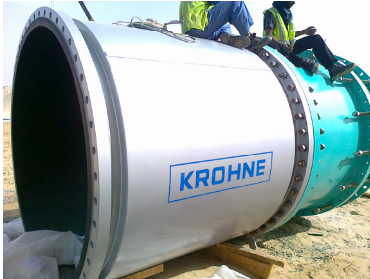
Figure 17 Inlet FM (prior to installation) had to be more accurate than usual for operating a wastewater plant, as the data from which was used as the basis for the monthly service payments.
