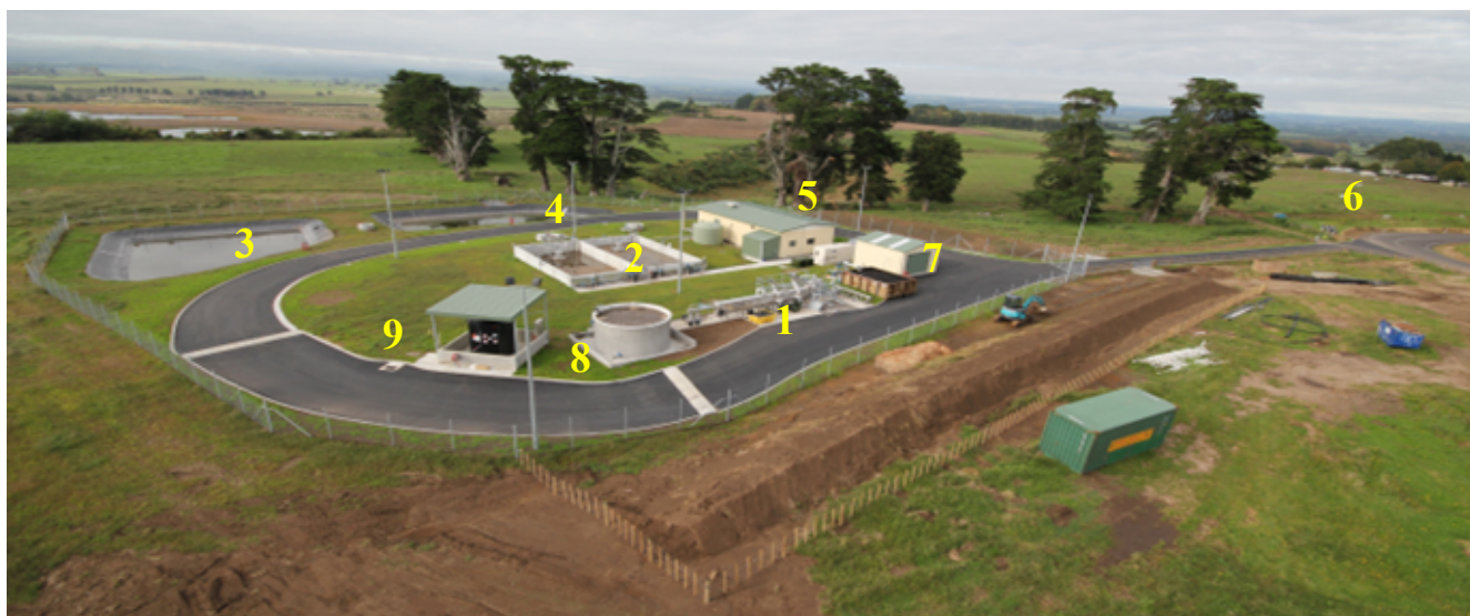
Photograph 6 – View of Maketu WWTP layout looking south west
