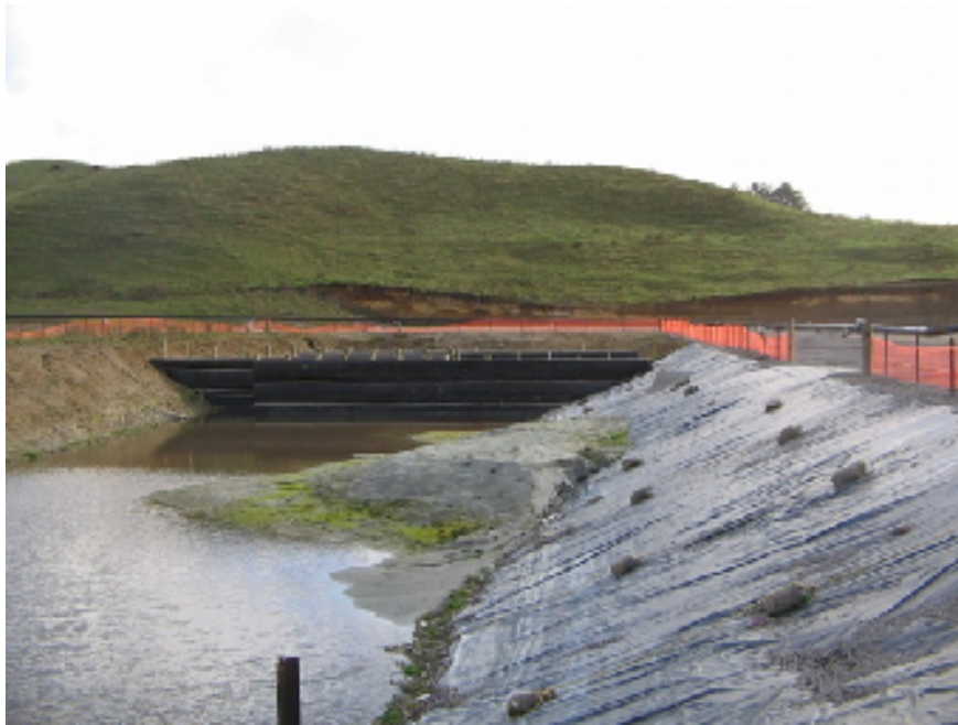
Photograph 1: Drained pond showing delta of cuttings.
