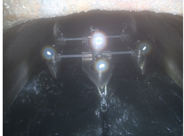
Photograph 2: "CCTV survey Boat to inspect pipes that are either flooded or under constant flow"
