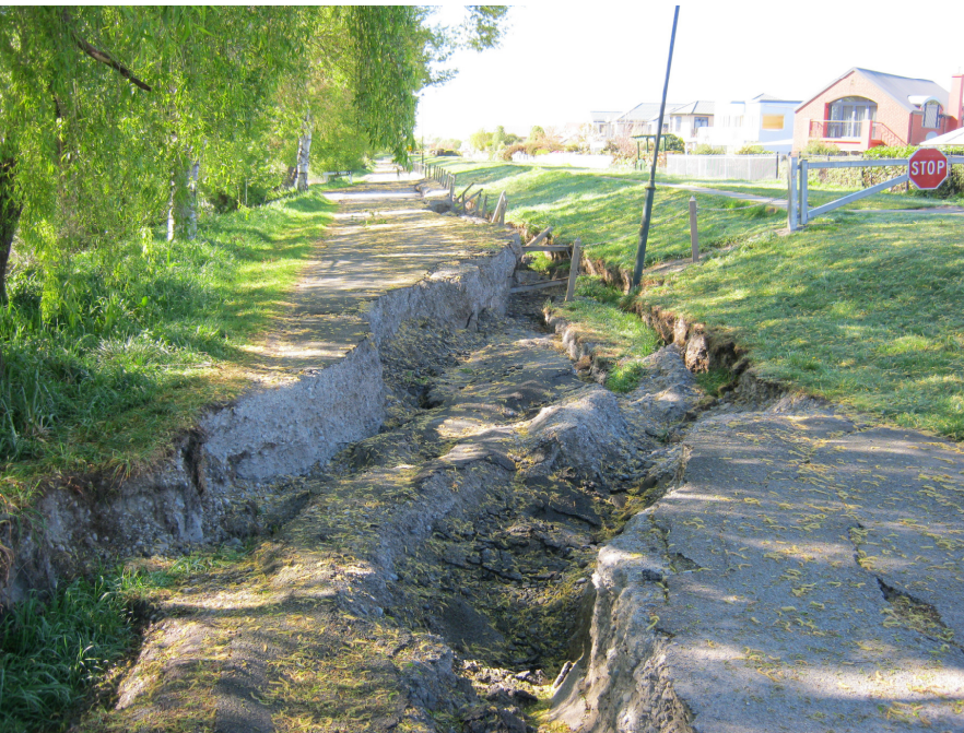
Figure 4: Lateral spread tension cracking on south side of Kaiapoi River adjacent to Bowler Street Stormwater pumping Station
