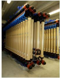
Banks of Pall Filters at the Taupo Water Treatment Plant capable of delivering up to 25,000 cubic metres of water per day.
