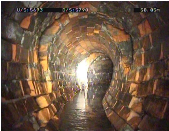
Figure 6 - Shear defect
