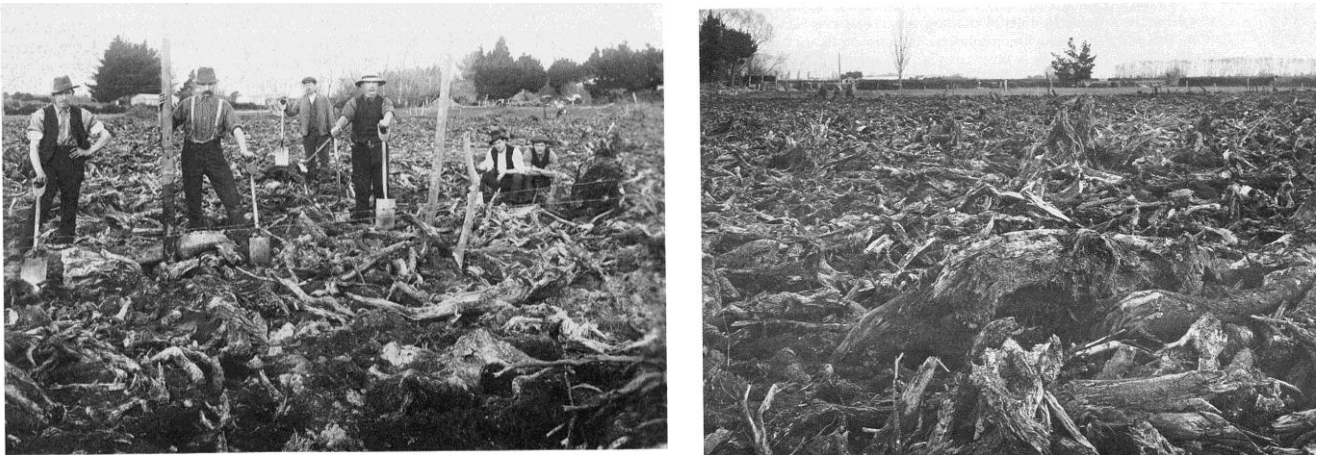
Figure 2 Construction conditions in 1918 (Christchurch Drainage Board)
