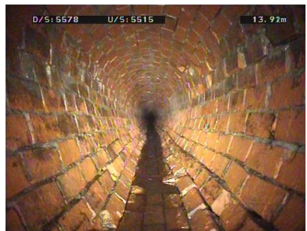
Figure 12 Effects of water blasting
