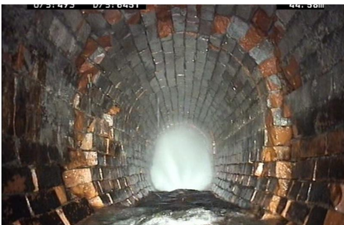
Figure 11 Flushing to remove silt by water jetting
