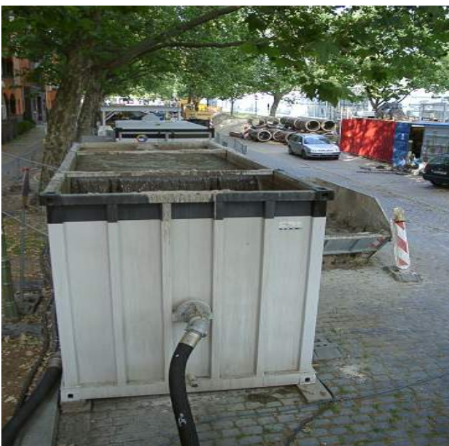
Photograph 2: Sediment Settling Tanks
