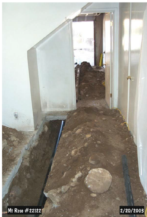
Photograph 4: Trenching through bedroom
