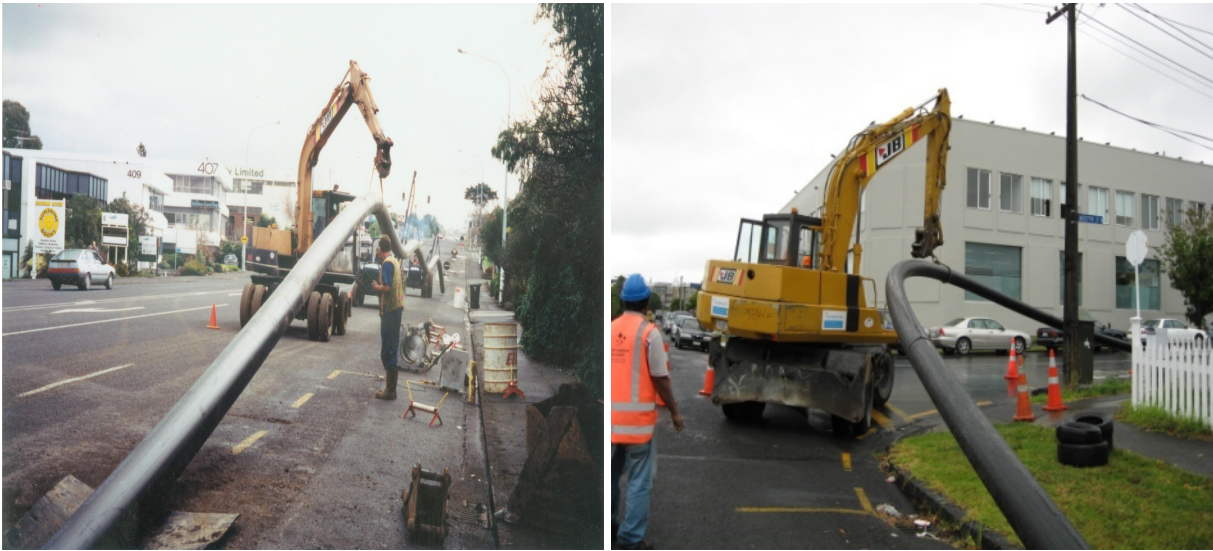
Photograph 1: Pipe Laydown Area
