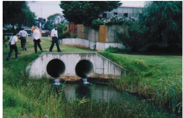
Photograph A5: Pipe(s) to pool
