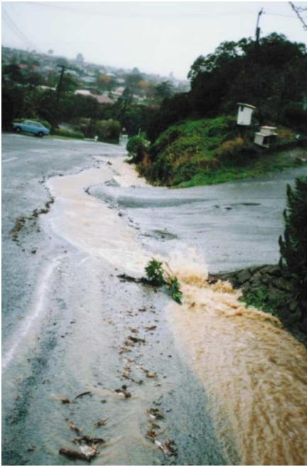
Photograph A7: Road drain to small culvert
