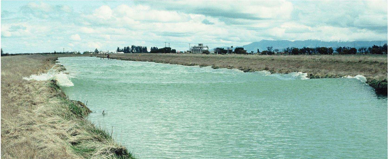
Photograph 2: Artificial Dambreak Surge, Rangitata Diversion Race
