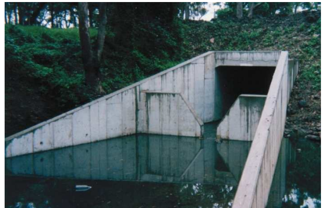
Photograph A6: Pool to V-Notch
