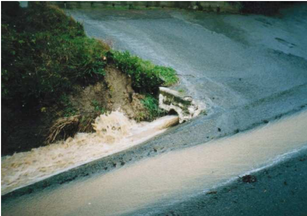
Photograph A8: Small culvert to road drain
