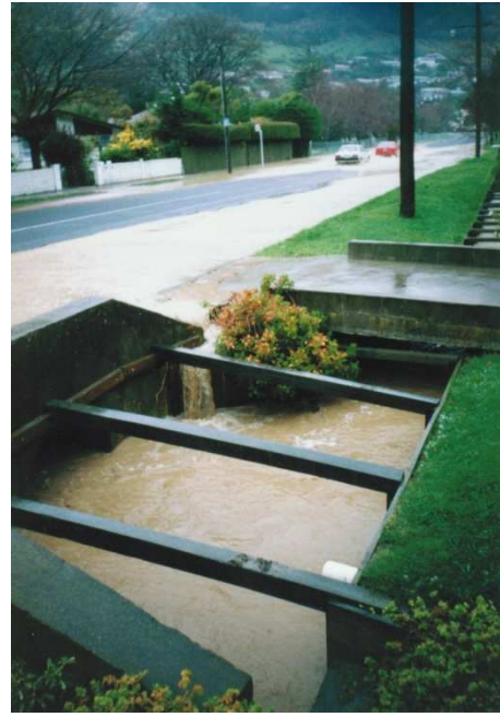
Photograph A9: Road Drain to large culvert
