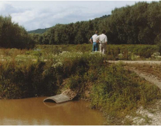
Photograph A2: Pool to pipe culvert
