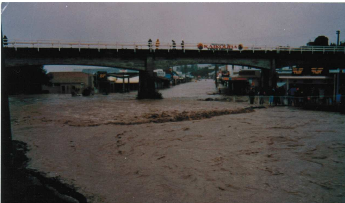
Photograph A11: Channel under bridge
