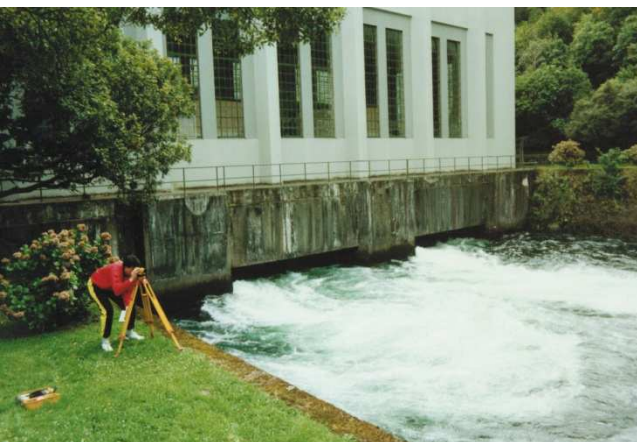
Photograph A3. Power station to channel
