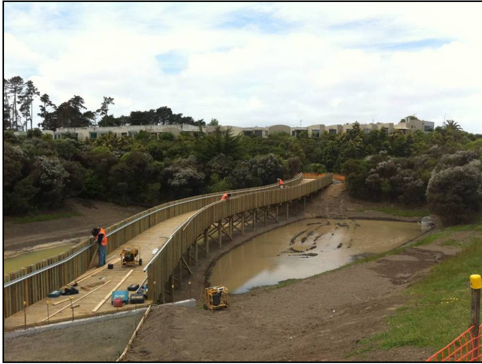
Figure 9: Cycleway Developed on top of the Separation Bund.
