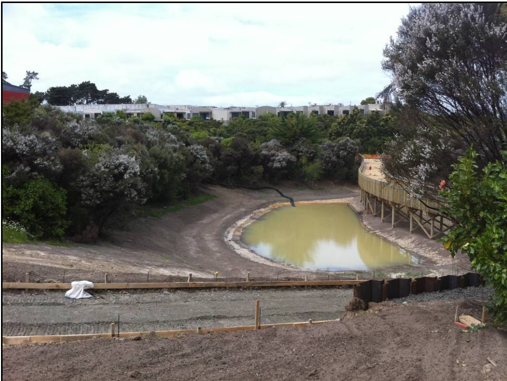
Figure 8: Omega Pond Showing Construction of Deep Water Forebay
