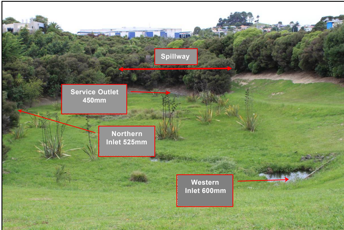
Figure 3: Showing Pre Works Omega Pond (facing East)
