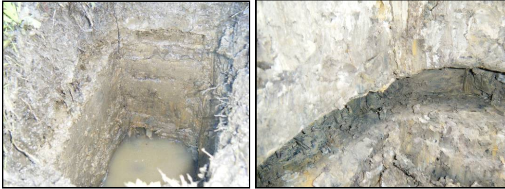
Figure 4: Showing Test Pits Dug into Accumulated Sediment
