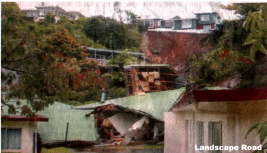
Photograph 1: Landslide at Otumoetai, Tauranga May 2005
