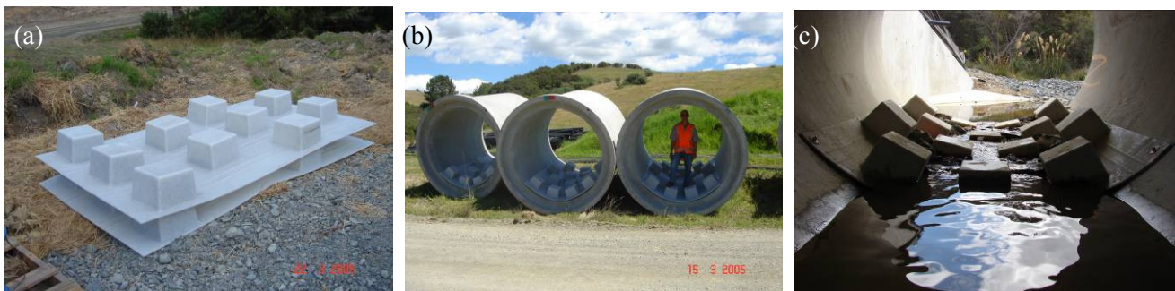
Photograph 3: Artificial riffles: a) plastic sheets as manufactured; b) placed in culverts and c) installed in culvert as riffles with matrix of natural materials.
