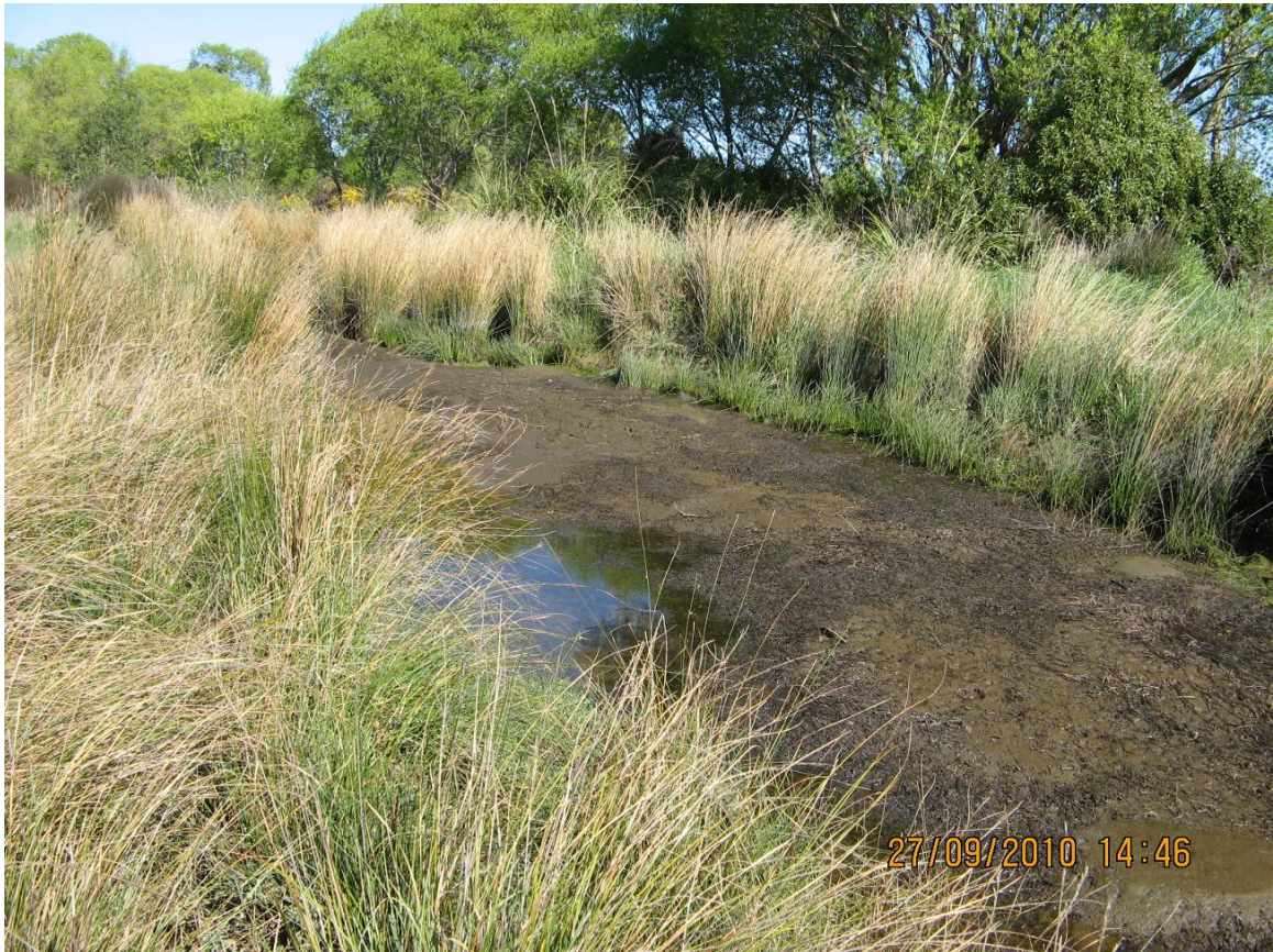
Photograph 2: Lower Styx Diversion Channel bed heave
