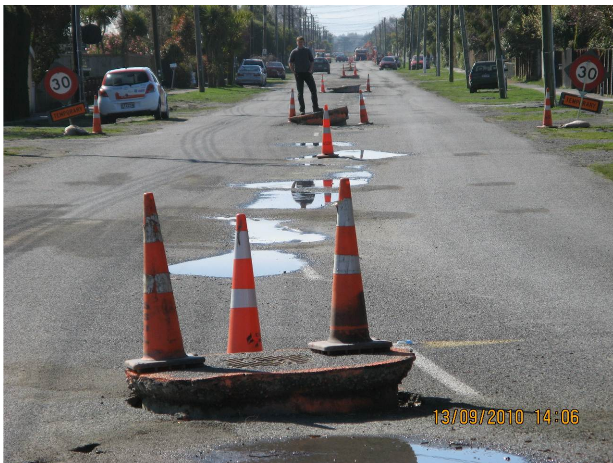
Photograph 3: Brooklands Sewer Manholes
