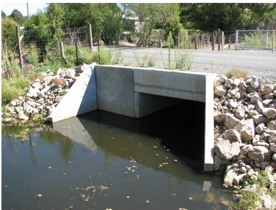
Photograph 5: Completed culvert construction
