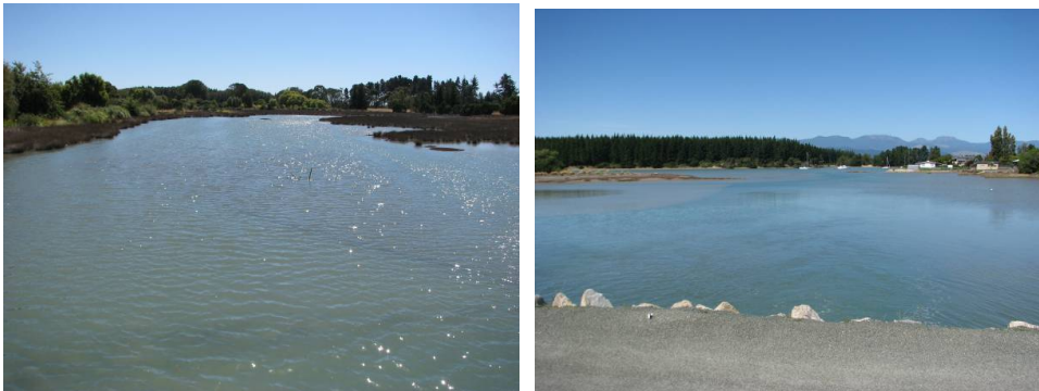
Photographs 1 and 2: Upstream and downstream Toru Street causeway
