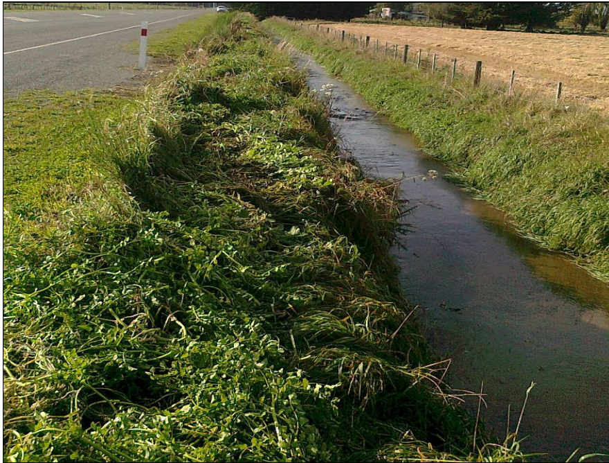
Picture 8: Drain cleaned with rake
