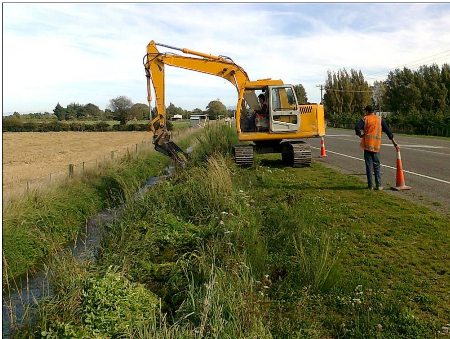
Picture 7: Cleaning with rake, weed is flicked onto edge of drain
