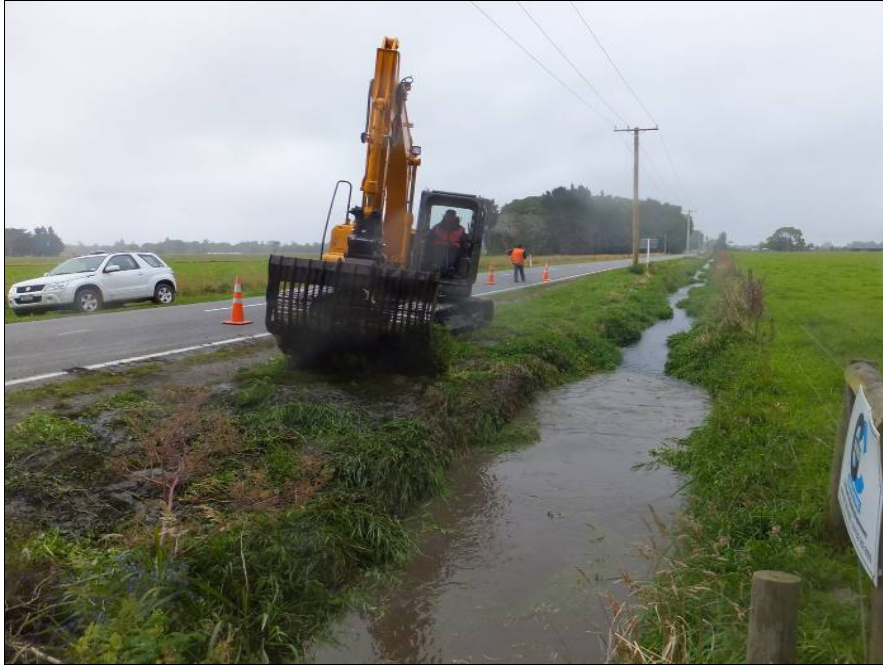
Picture 4: Cleanings placed alongside drain
