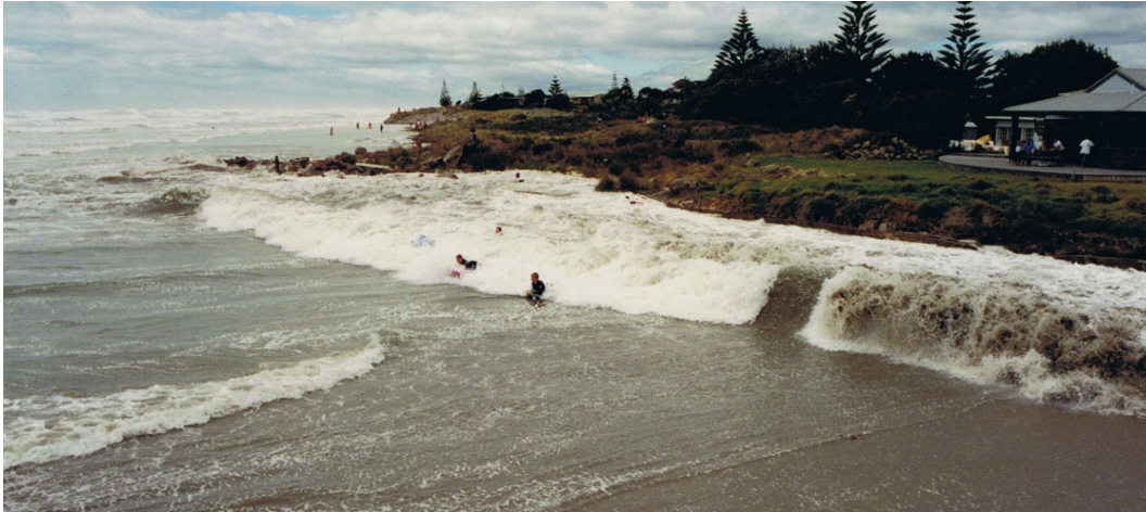
Photograph 4: Two Mile Creek mouth prior to coastal protection works
