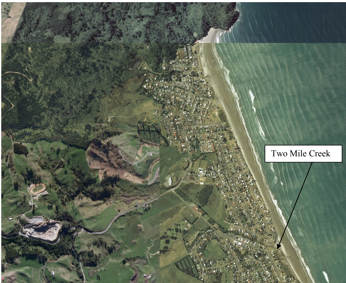
Photograph 3: Waihi Beach – 2008 (copyright Terraview)
