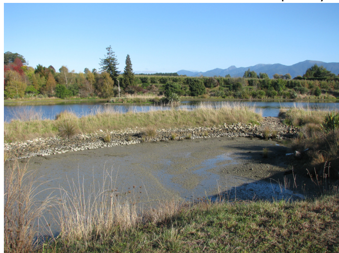
Figure 3: Example of a passive weir built to maintain fresh water levels for irrigation in the background while the tidal zone enters the foreground up to the rocks. A concrete overflow is to the right of the passive weir structure.
