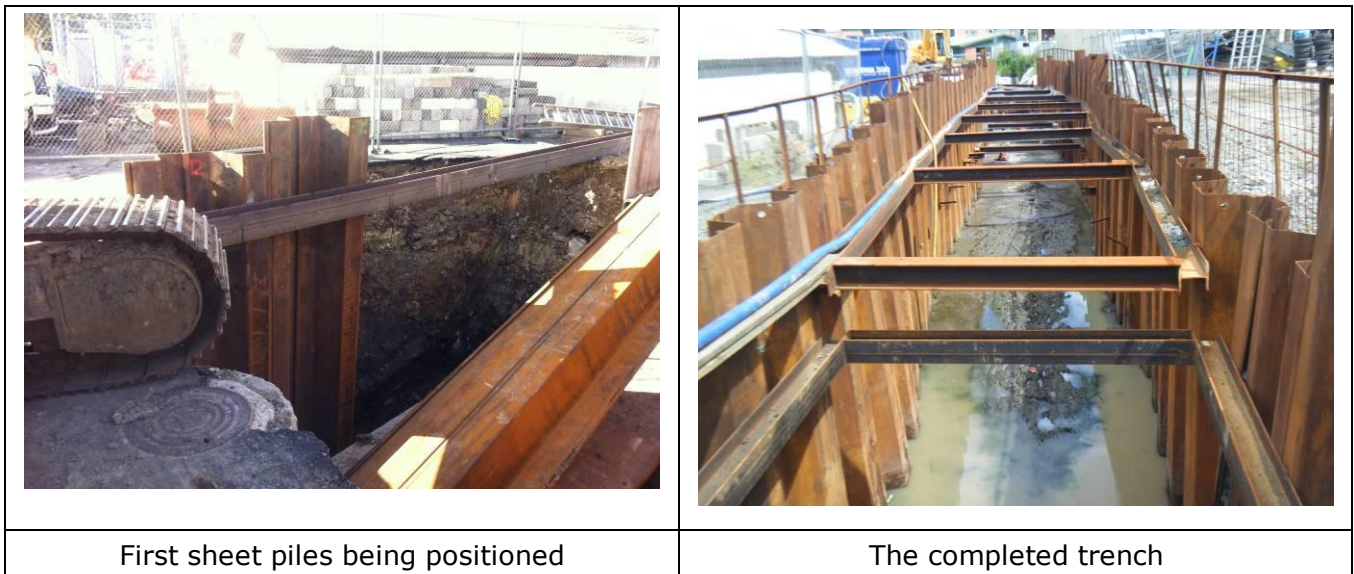
Photograph 4: Excavated trench showing sheet pile shoring
