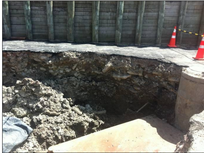
Photograph 2: Photo showing uncontrolled fill within 3 Cartwright Road
