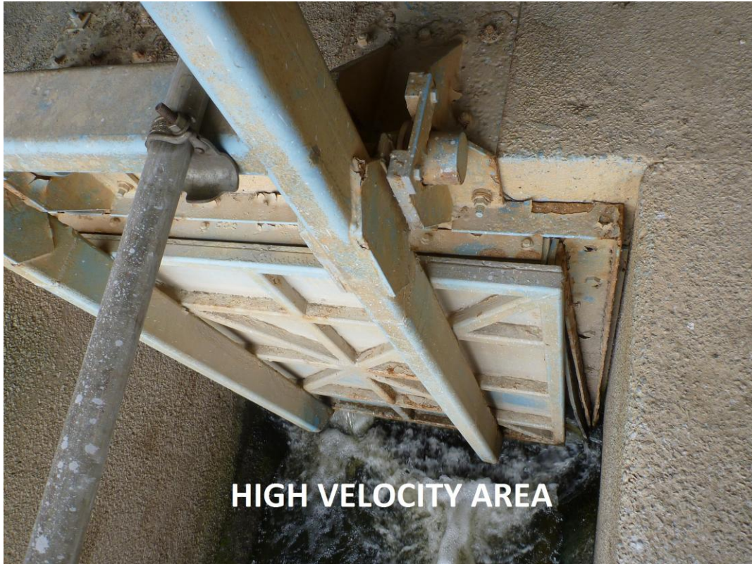
Photo 3: Looking down on to gravity flapgate
