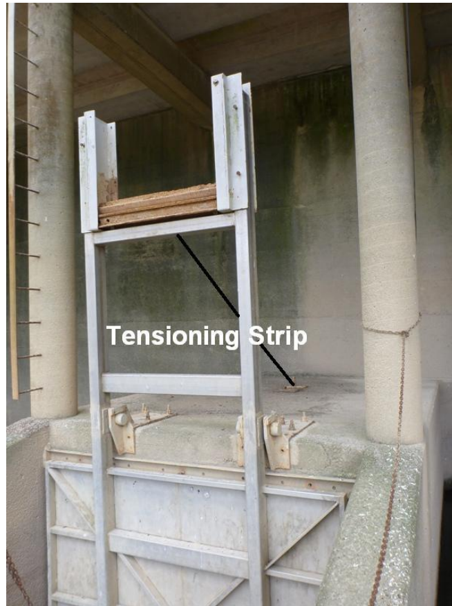
Photo 5: Tensioning strip to keep gate partially open
