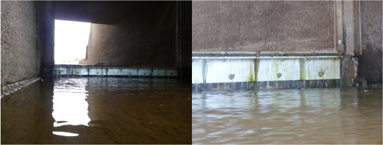
Photo 4: Looking upstream to gravity flapgates & overhang
