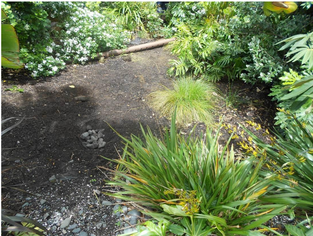
Photograph 1: Maintenance access to raingarden is restricted
