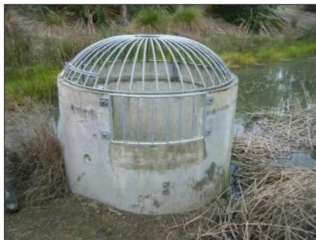
Photograph 68: Showing Outlet Configuration
