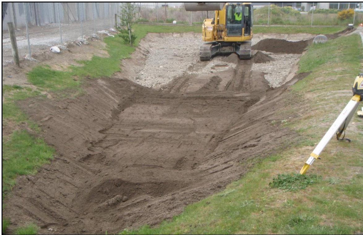
Figure 5: Basin infiltration media being placed
