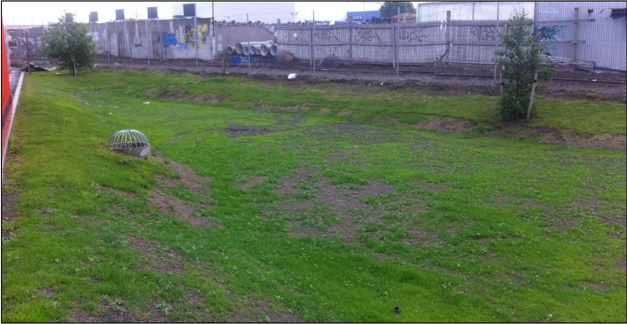
Figure 6: Infiltration basin 1 month after remediation
