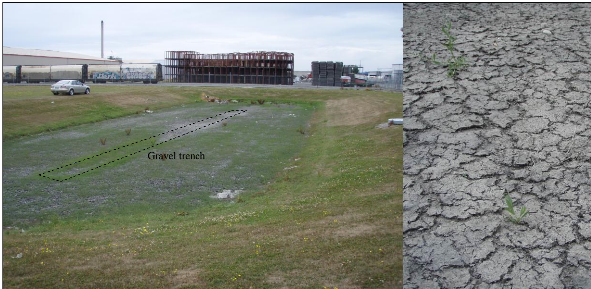
Figure 12: Basin after installation of trench
