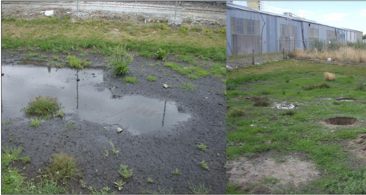
Figure 2: Infiltration basin after topsoil replaced
