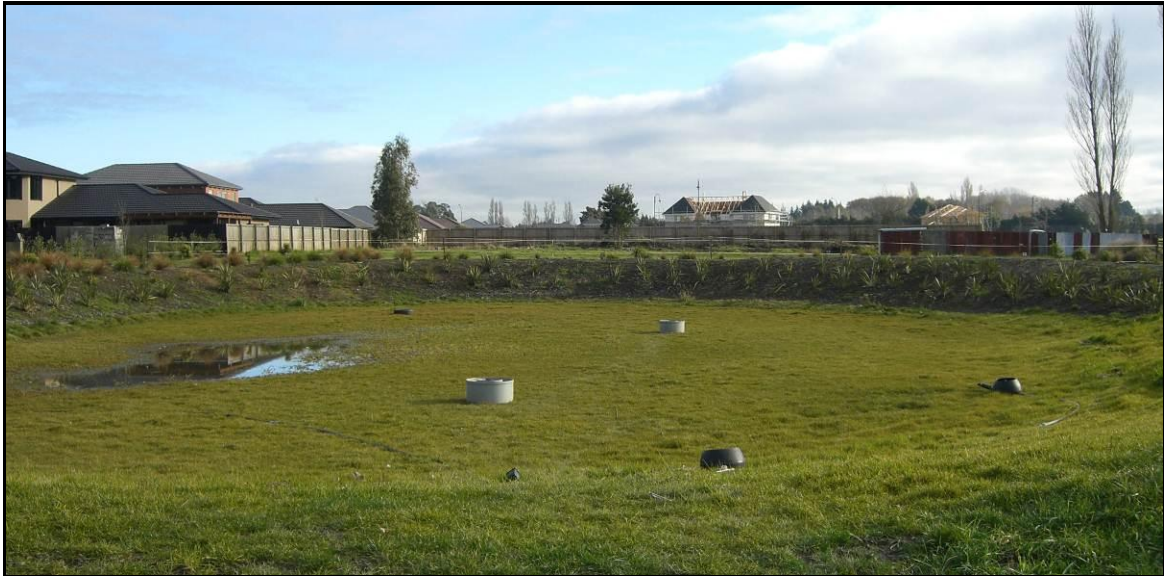
Figure 7: Basin after installation of trench
