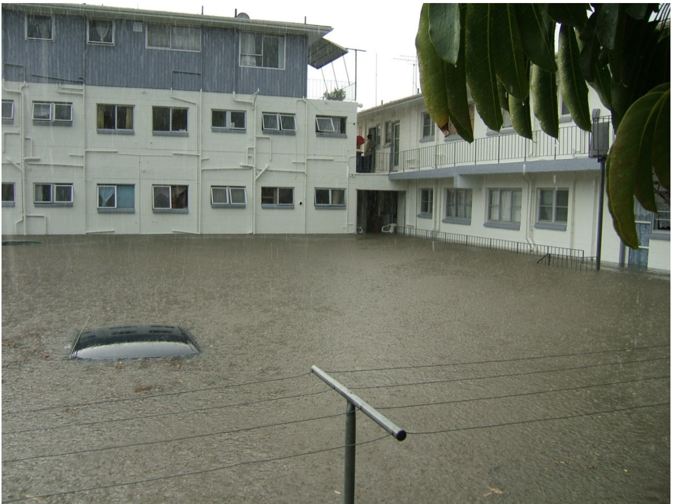
Figure 11: Cartwright Road flooding
