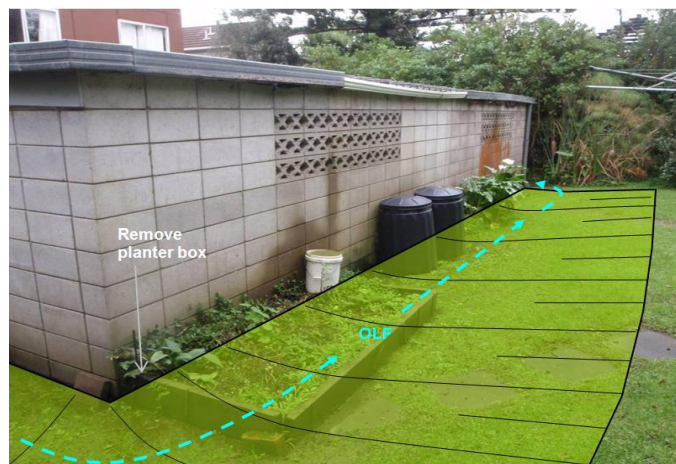
Photograph 4: Landscape and contour land to form overland flow path
