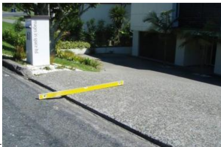
Photograph 1: Driveway crossing with inadequate roll over
