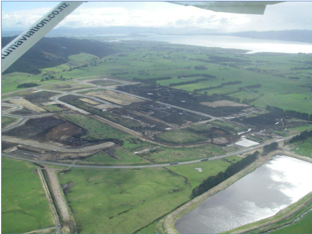
Figure 1: Marsden City & 6ha wet pond – construction monitoring aerial photograph 2009
