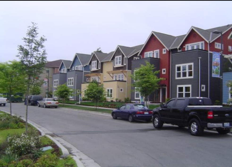
Social housing development in Seattle (photo 2006 | name Highpoint
