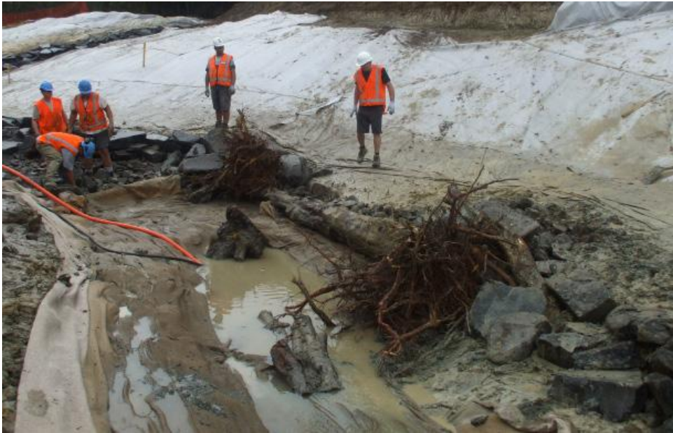
Figure 8: Rootwads and woody debris integrated with rock for slope-toe protection
