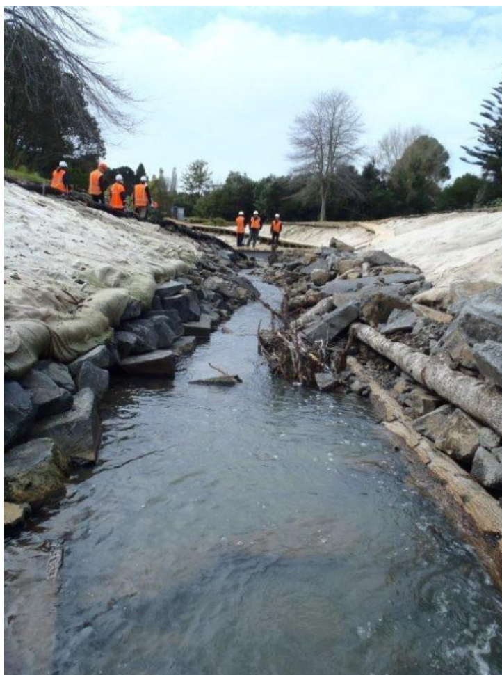
Figure 9: Rock and woody debris integrated with soil lifts, compost socks, and wool mat
