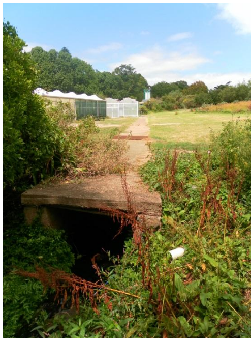
Photograph 3: View upstream showing the box culvert (source: Estrin, 2013)
